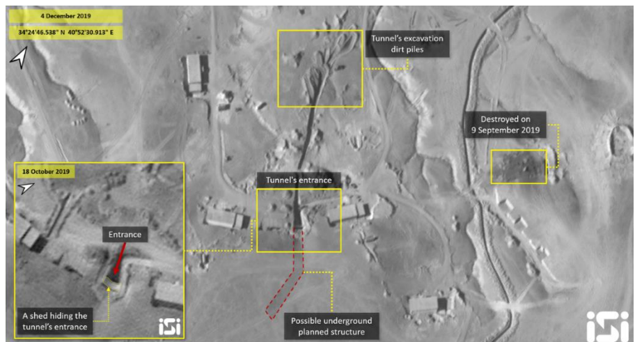
Image no.10: New tunnel-digging in the Imam Ali military base in Al Bukamal.
